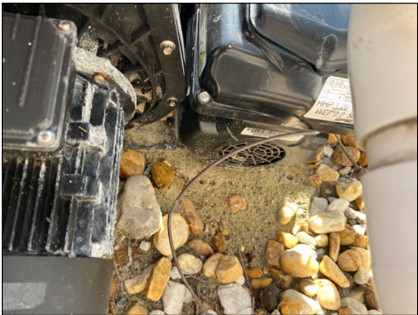
Bonding in place and appears functional
