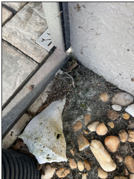
Bonding in place and appears functional
