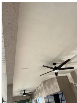
Loose soffit on front porch. Recommend having re-secured. Front patio
