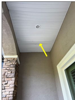
Loose soffit on front porch. Recommend having re-secured. Front patio
