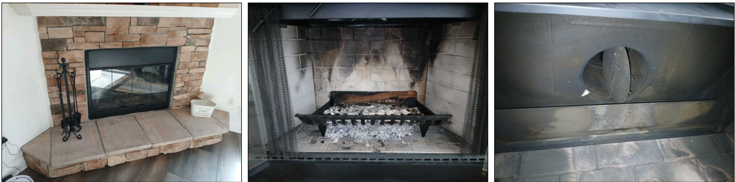
Damper was opened and closed several times.
