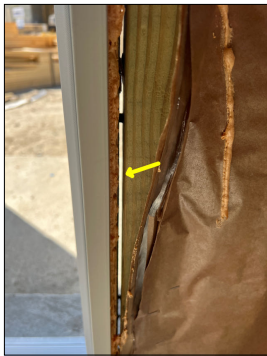
Front door not properly sealed.
