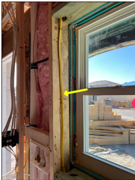
Wires need moved into wall cavity.
