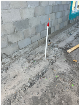
Condensate drip line outside HVAC closet, this is in the living space area. Recommend builder evaluate and repair. Condensate drip line outside HVAC closet, this is in the living space area. Recommend builder evaluate and repair.
