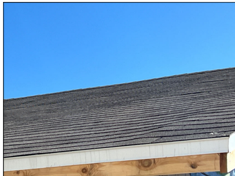
Several shingles curling/lifting noted.
