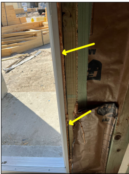
Front door not properly sealed.
