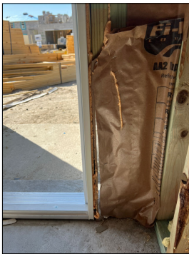
Front door not properly sealed.
