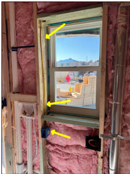
Wires need moved into wall cavity.
