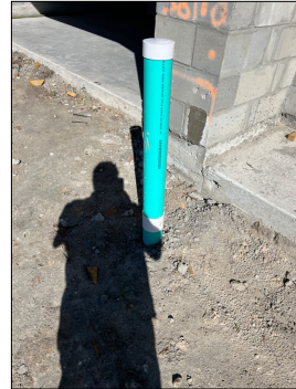
PVC sewer drain pipes found properly plugged and holding water at the time of inspection.
