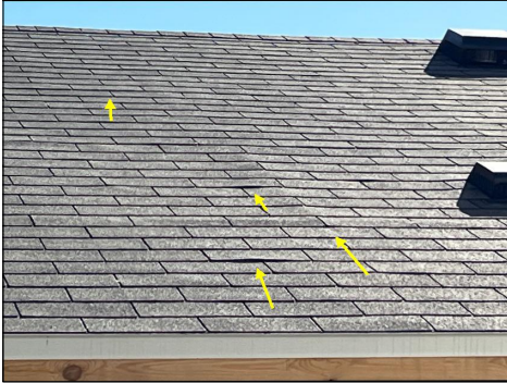
Several shingles curling/lifting noted.
