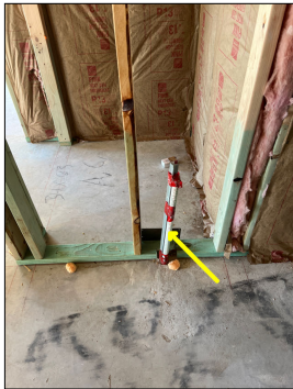
Condensate drip line outside HVAC closet, this is in the living space area. Recommend builder evaluate and repair. Condensate drip line outside HVAC closet, this is in the living space area. Recommend builder evaluate and repair.
