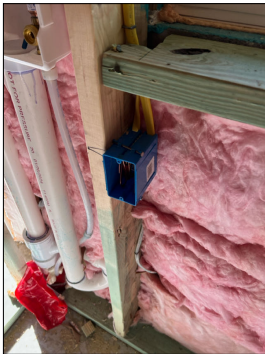
Wires need moved into wall cavity.
