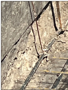
Ground wire installed.
