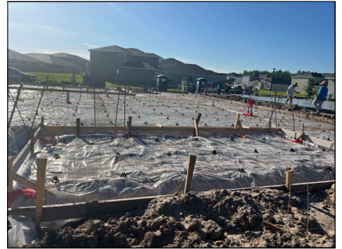
Fix vapor barrier not fully extended under footers to outer edge of slab.
