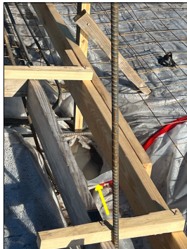
Fix vapor barrier
