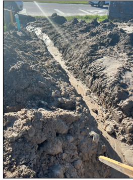
Main sewer line not installed.
