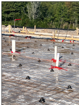
Supply lines not pressurized at the time of inspection, inspector noted zero psi, recommend builder evaluate. FBC 2503.7. No Gauge found on property.
