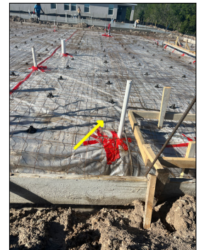
Several missing chair rails seats under wire mesh.
