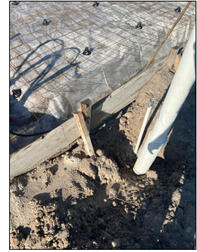
Main sewer line not installed.
