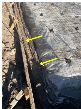
Fix vapor barrier not fully extended under footers to outer edge of slab.
