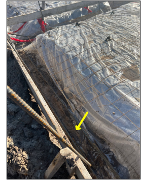
Fix vapor barrier not fully extended under footers to outer edge of slab.
