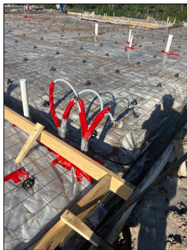
Supply lines not pressurized at the time of inspection, inspector noted zero psi, recommend builder evaluate. FBC 2503.7. No Gauge found on property.
