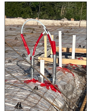
Supply lines not pressurized at the time of inspection, inspector noted zero psi, recommend builder evaluate. FBC 2503.7. No Gauge found on property.
