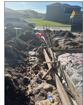
Supply lines not pressurized at the time of inspection, inspector noted zero psi, recommend builder evaluate. FBC 2503.7. No Gauge found on property.
