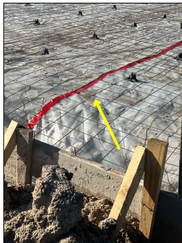
Several missing chair rails seats under wire mesh.
