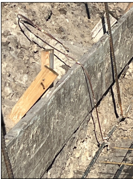
Ground wire installed.
