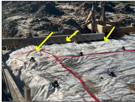
Several missing chair rails seats under wire mesh.
